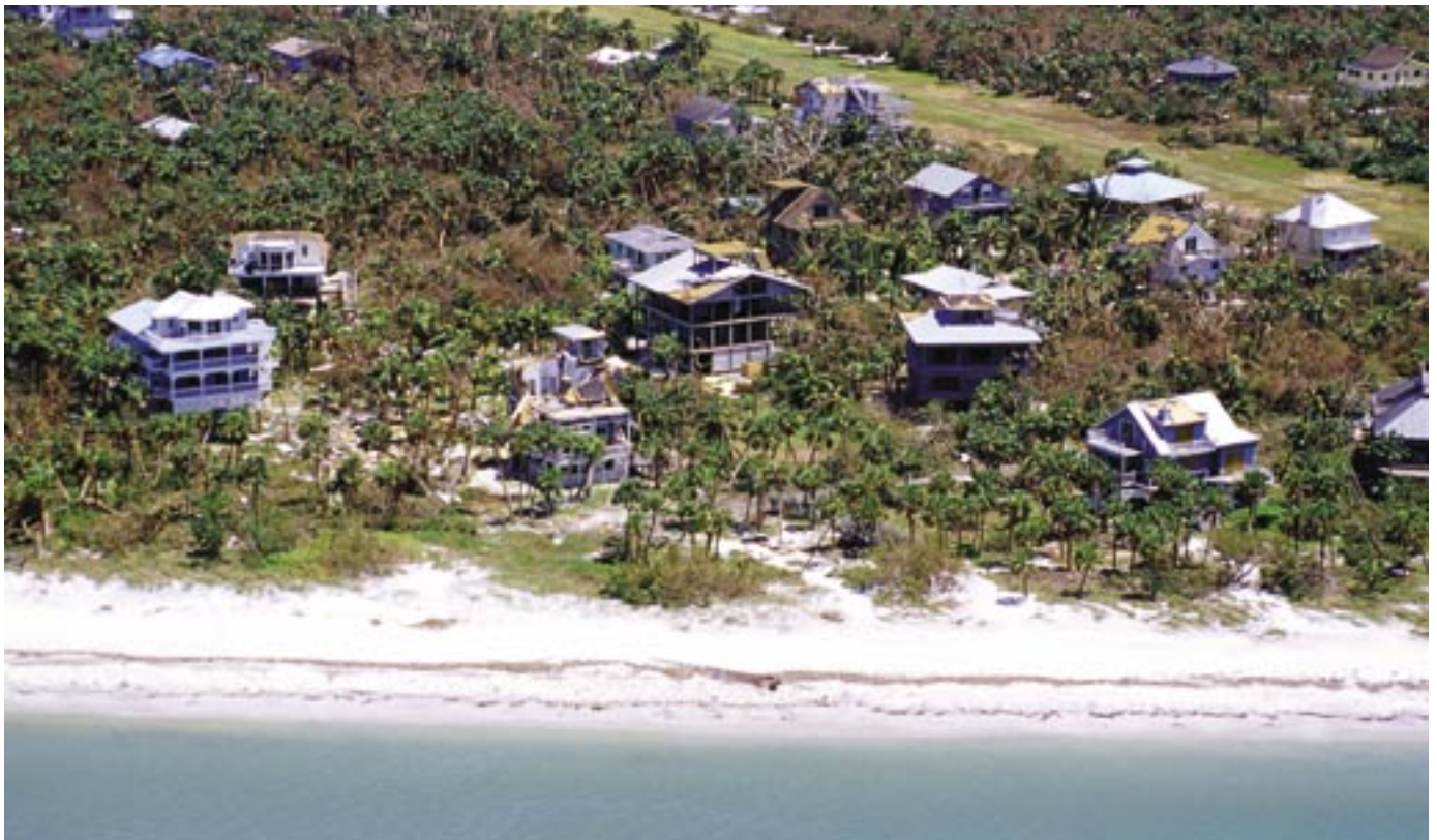
Damage to homes from Hurricane Charley in North Captiva
